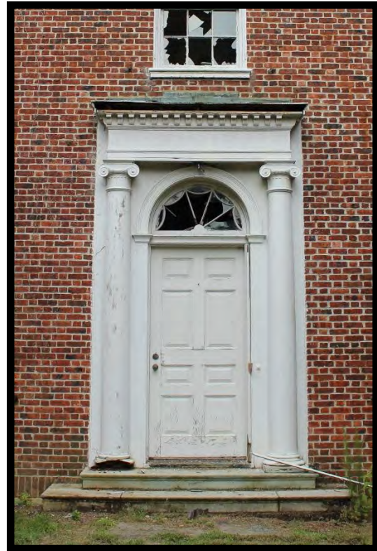
Figure 5: Entry Door, Merriemeade, Looking West.
