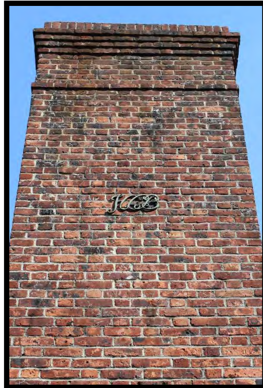
Figure 7: Chimney Detail, Merriemeade, Looking North.
