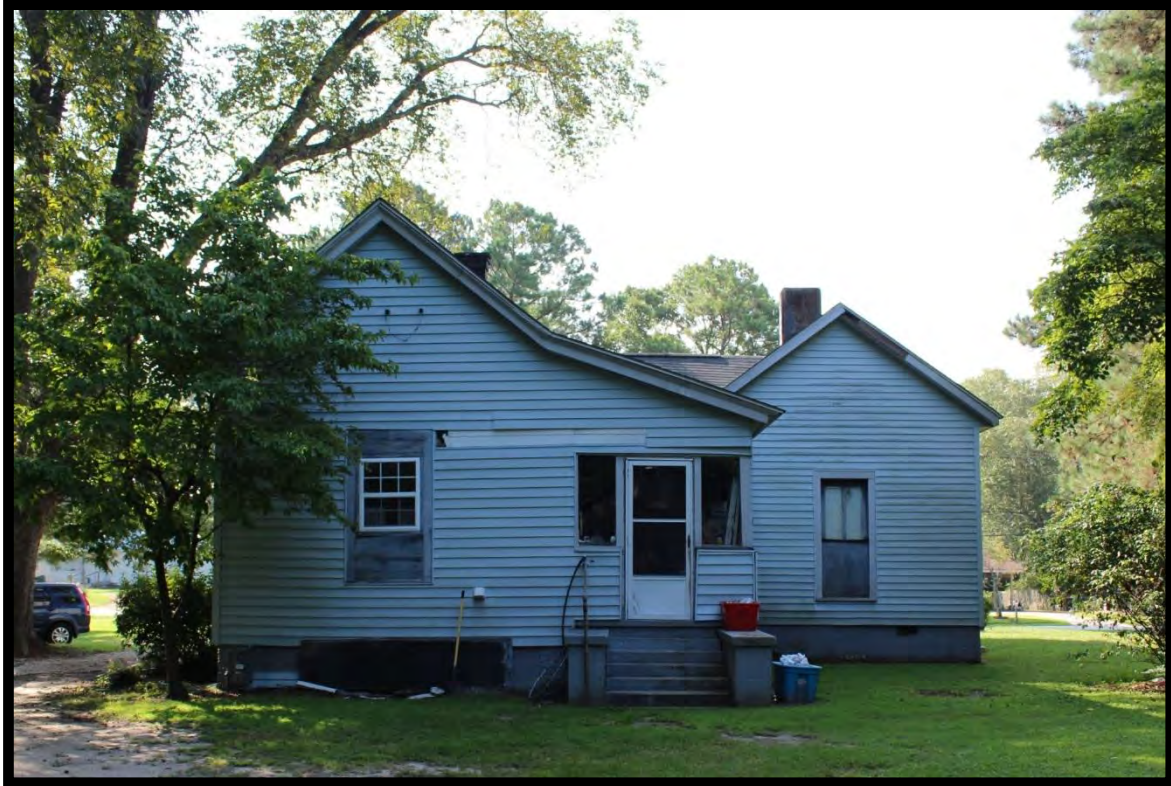
Figure 36: Johnston House, Looking Southeast.
