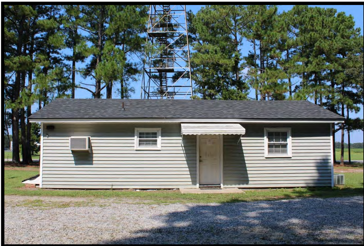
Figure 103: Office, Fire Lookout Tower, Looking Northwest. Note fire tower in background of photo.
