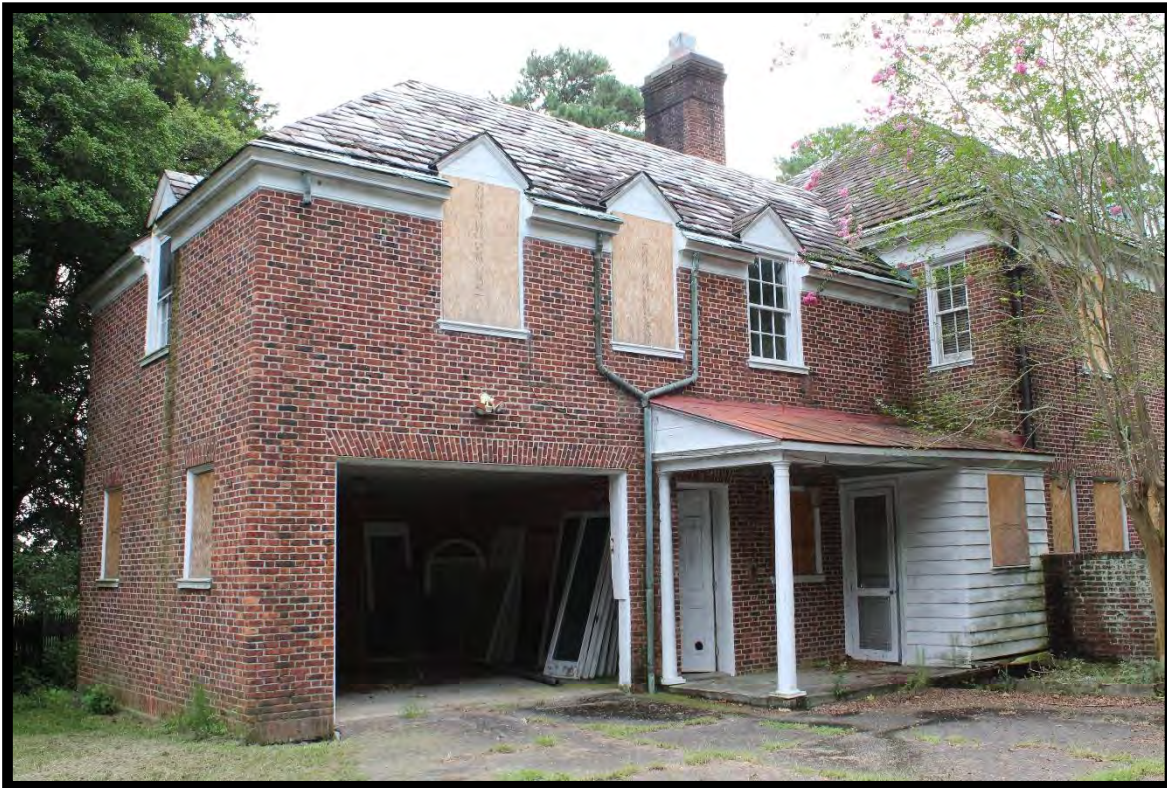
Figure 11: Window Detail, Merriemeade, Looking West.
