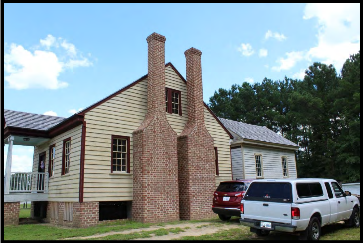
Figure 71: Norfleet House, Looking East.
