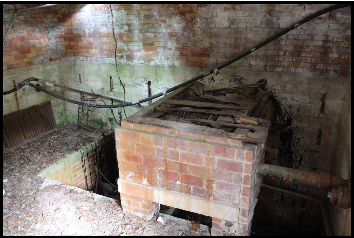
Figure 22: Interior of Cistern.
