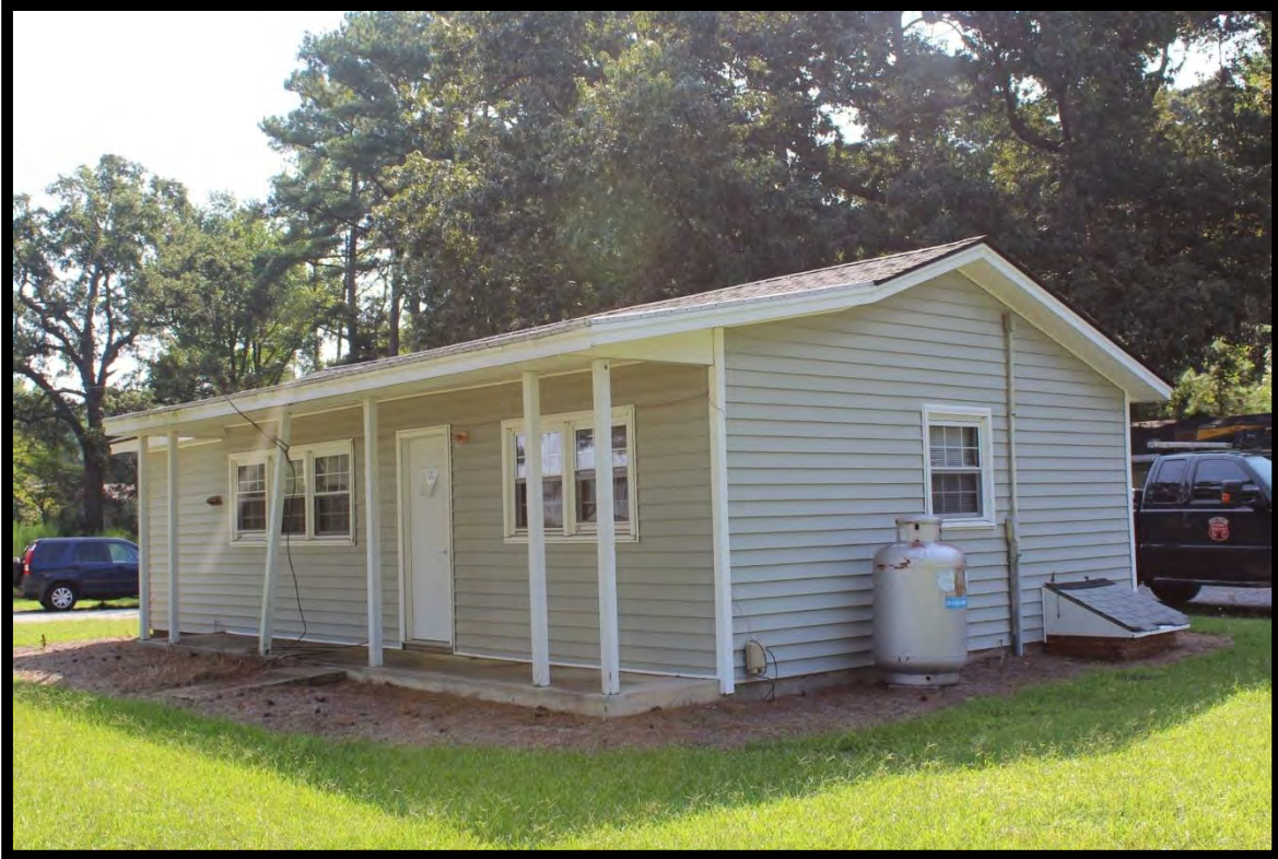
Figure 102: Office, Fire Lookout Tower, Looking East.
