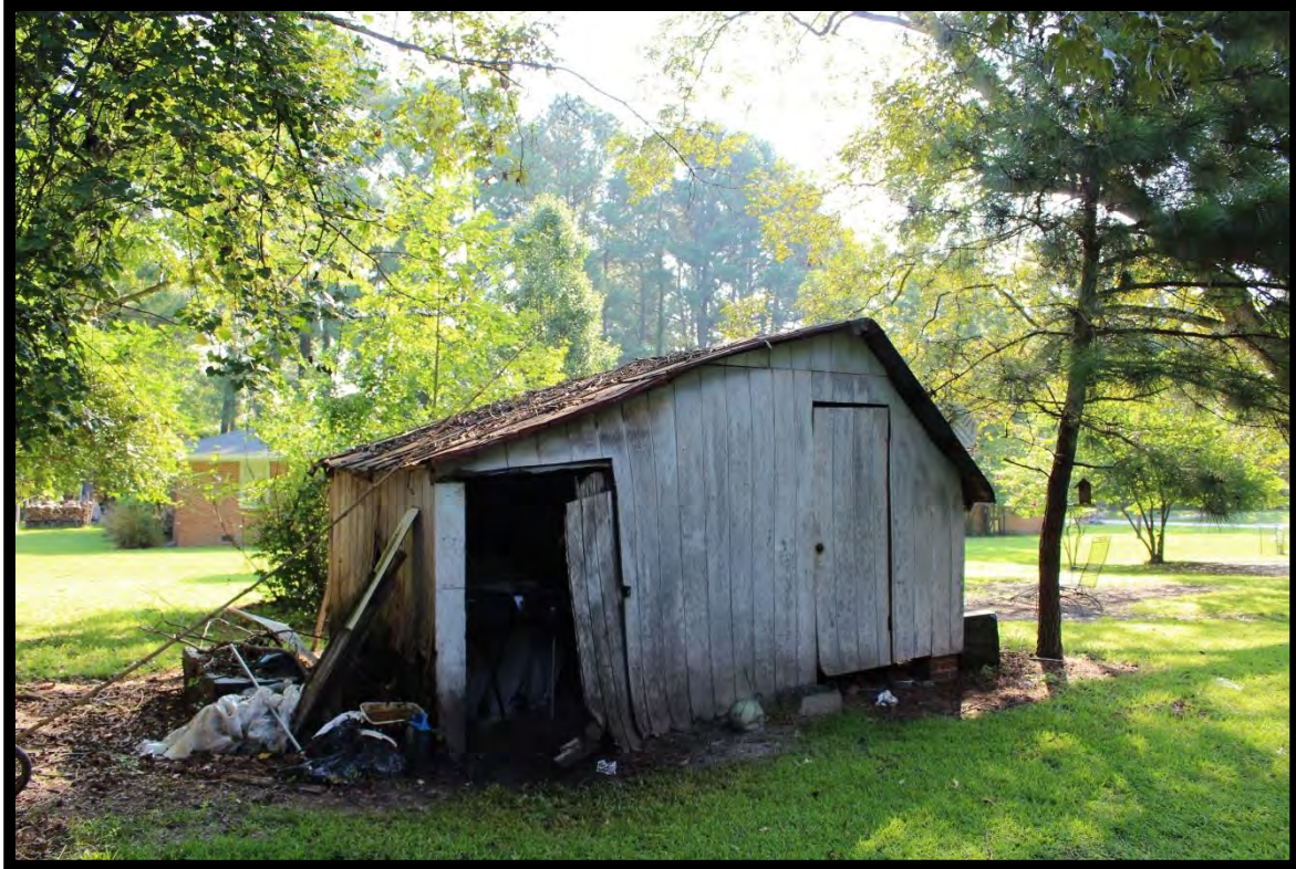
Figure 40: Shed, Looking East.
