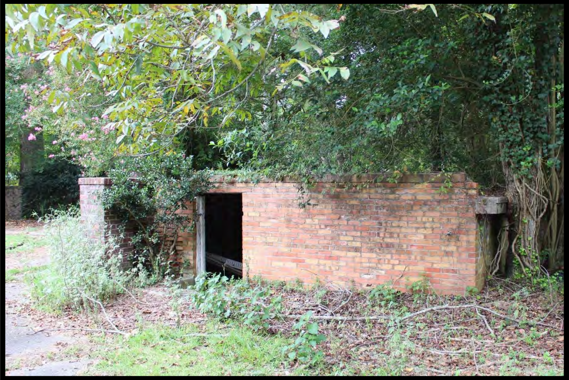
Figure 21: Cistern, Looking Southwest.
