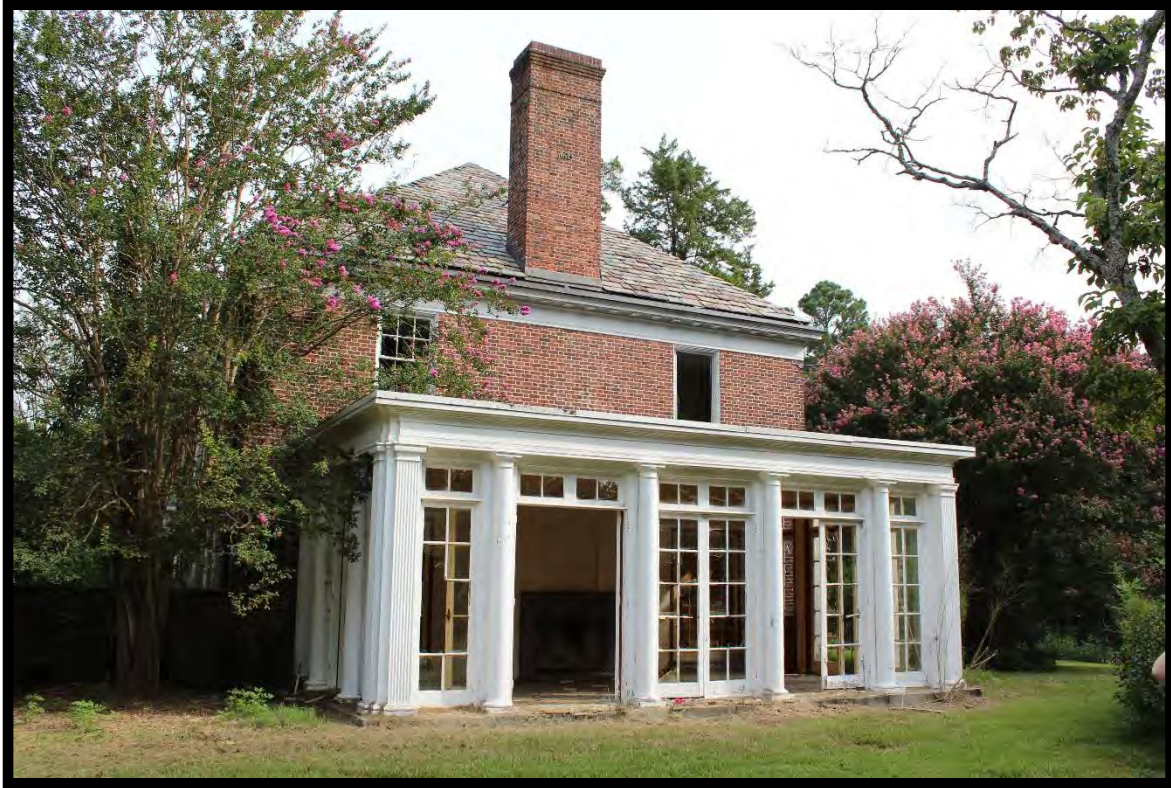
Figure 6: Merriemeade, Looking Northeast.
