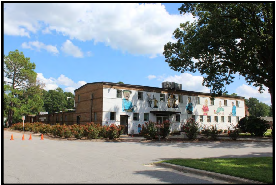
Figure 93: Former Edgecombe County Prison Camp Building, Now Used by Edgecombe Community College.
