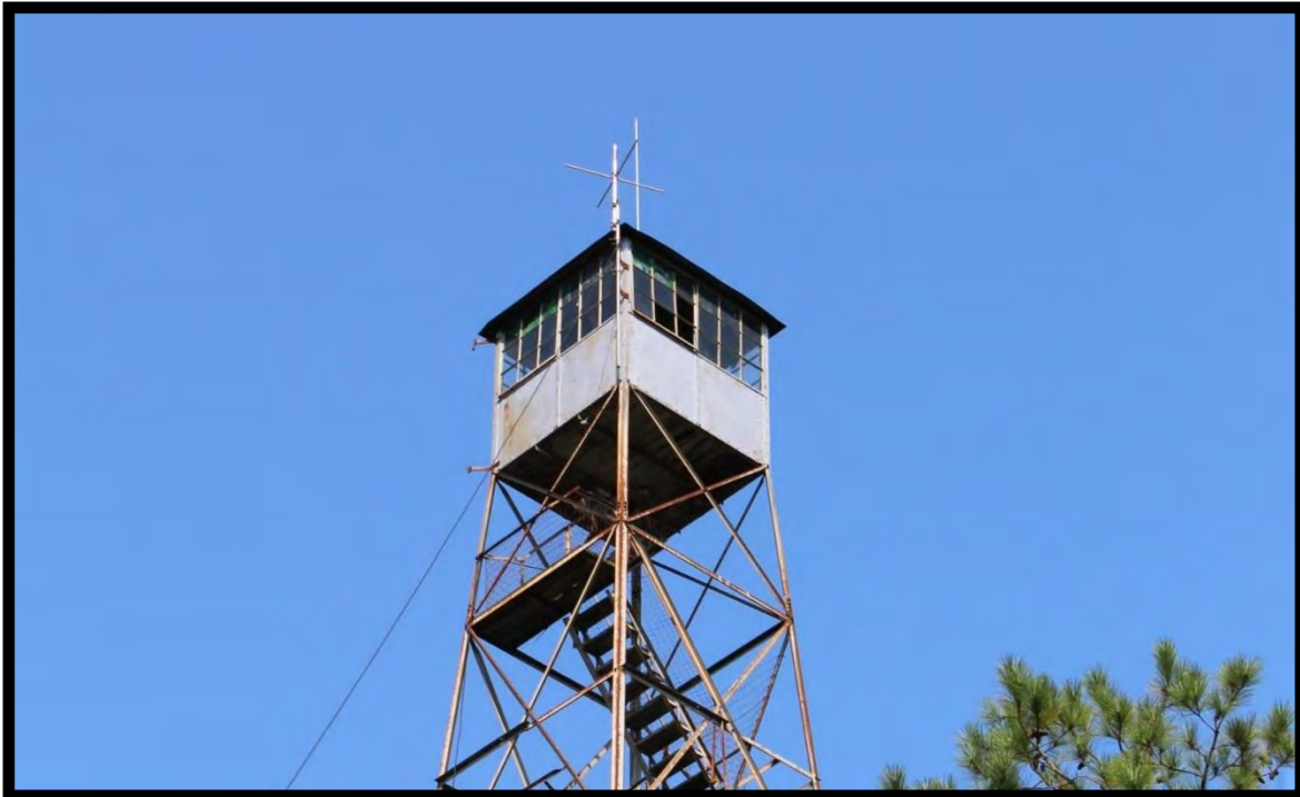
Figure 101: Fire Lookout Tower, Looking West.
