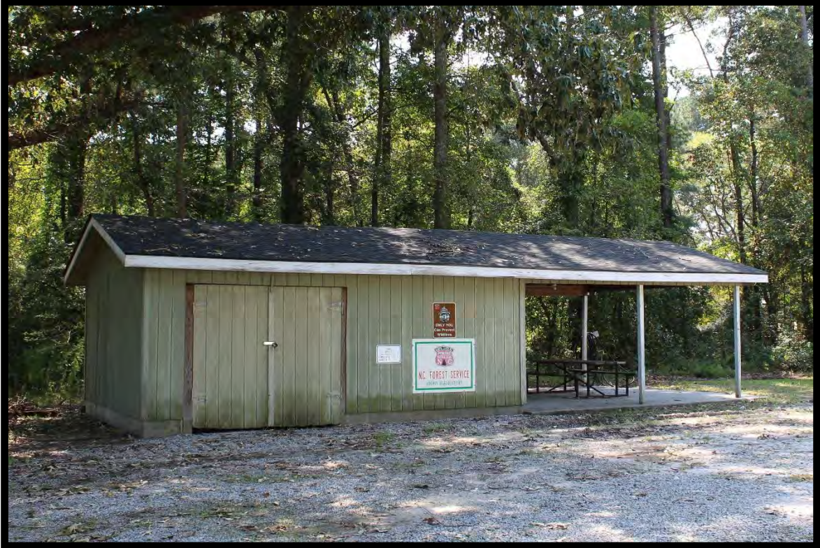
Figure 104: Shed, Fire Lookout Tower, Looking South.
