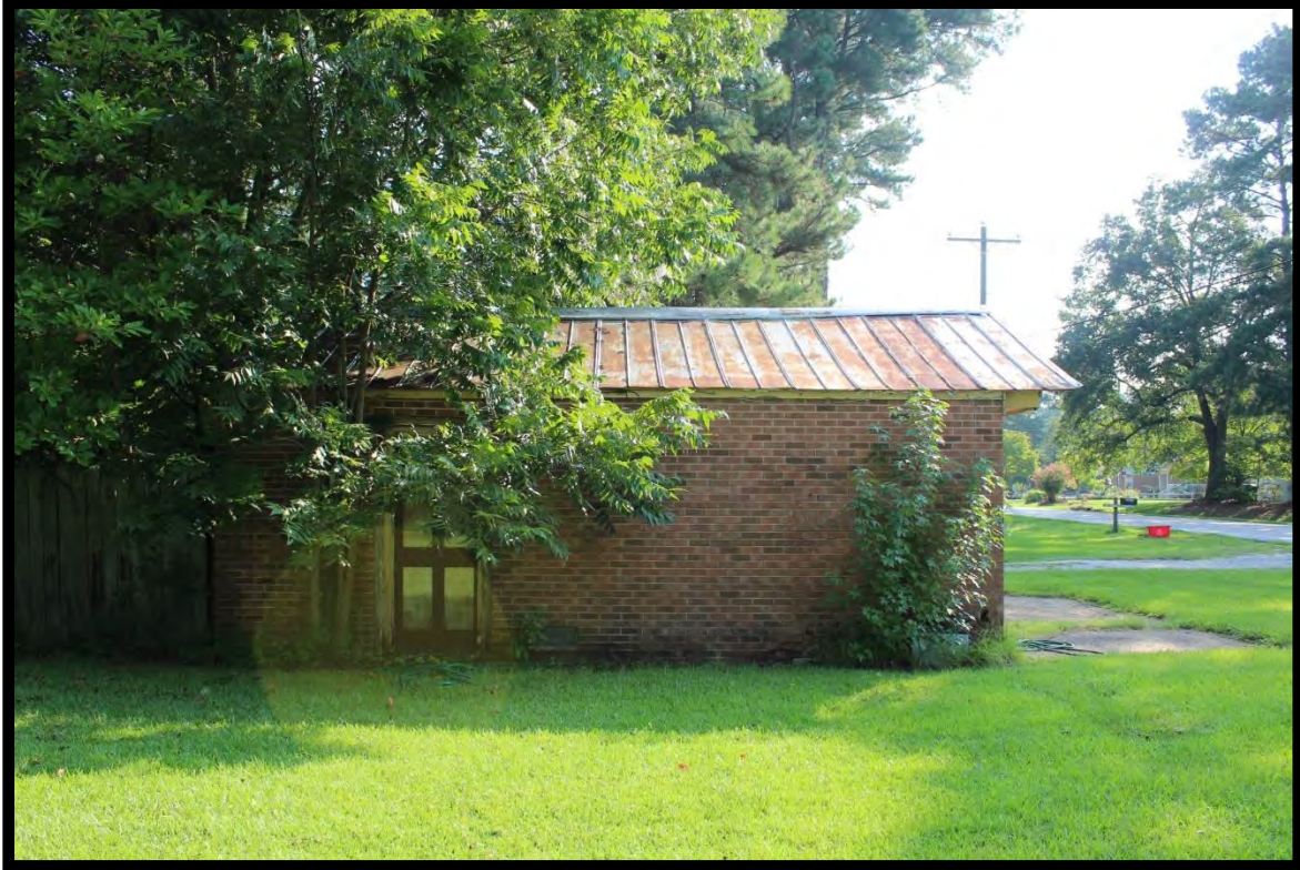
Figure 45: Store, Looking Northeast.
