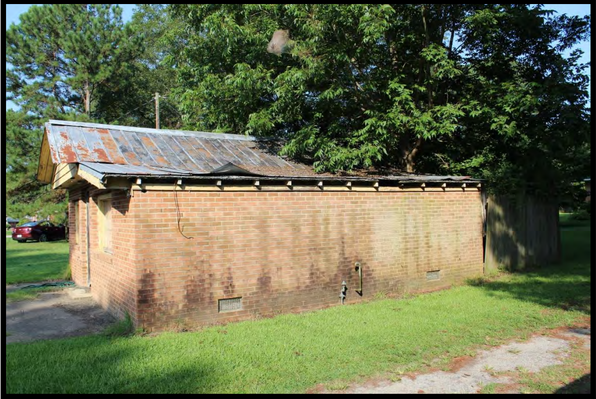
Figure 43: Store, Looking East.
