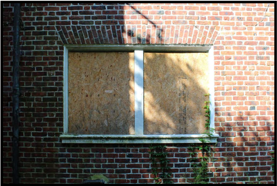
Figure 9: Window Detail, Merriemeade, Looking West.
