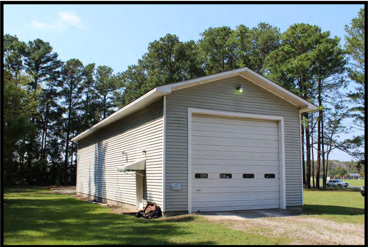
Figure 105: Equipment Shelter, Fire Lookout Tower, Looking West.
