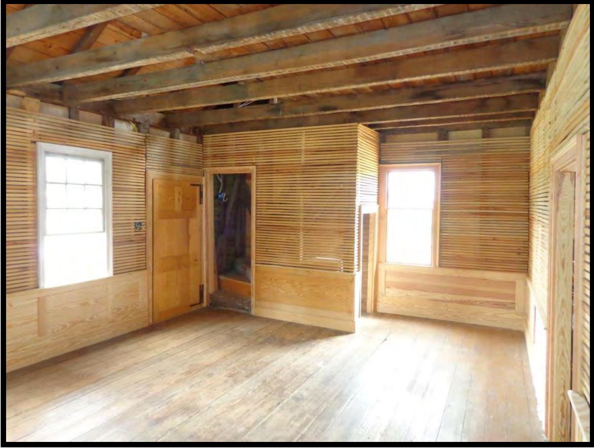
Figure 95: Norfleet House During Restoration (Monika Fleming).
