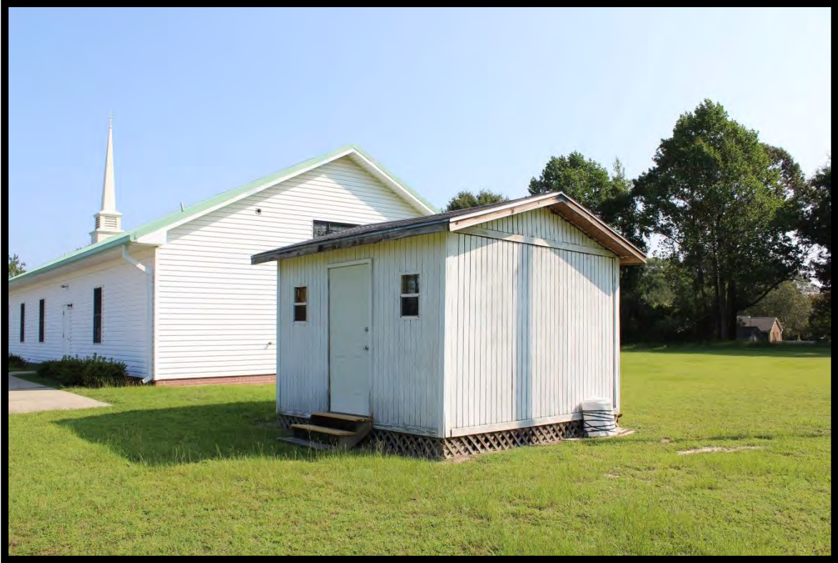
Figure 59: Shed, Looking Northeast.
